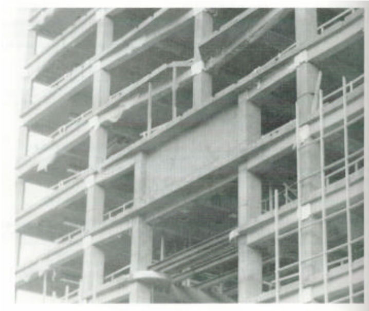
Fig. 1-1 Transfer girder [1].
