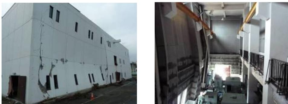
Fig. 1.14 Three-story RC wall-frame building damaged by tsunami [57]
