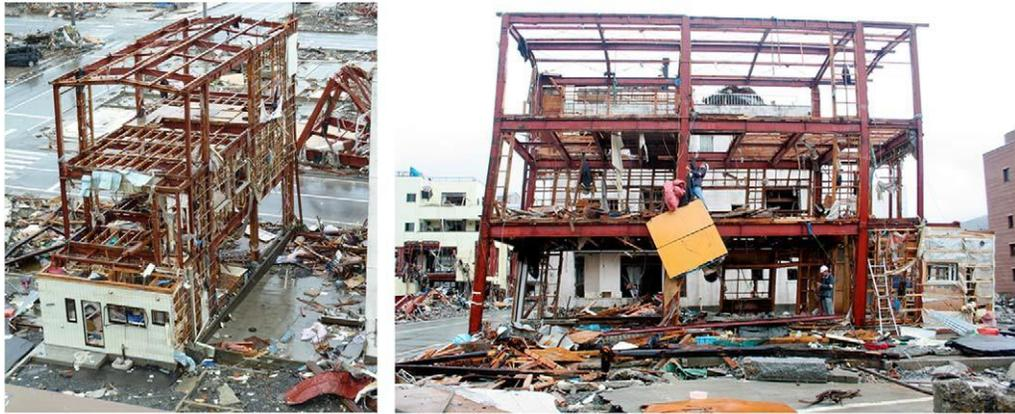
Fig. 1.15 A three-story steel-frame building damaged by tsunami [56]
