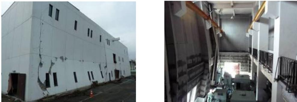
Fig. 2.14 Damage of a three-story RC wall-frame building [57]
