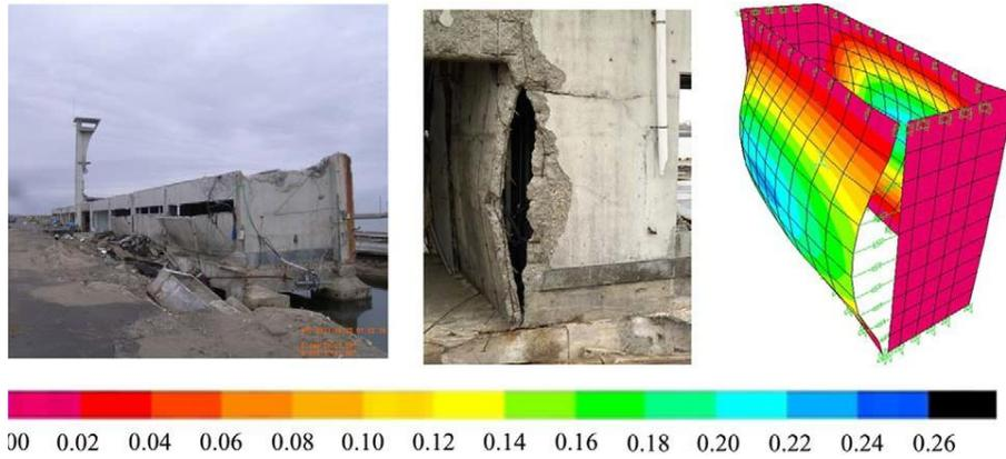
Fig. 1.16 FEM analysis of a large fish market building damaged by tsunami [56]
