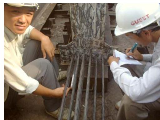
Fig.5.2.5: Measurement of strand elongation
