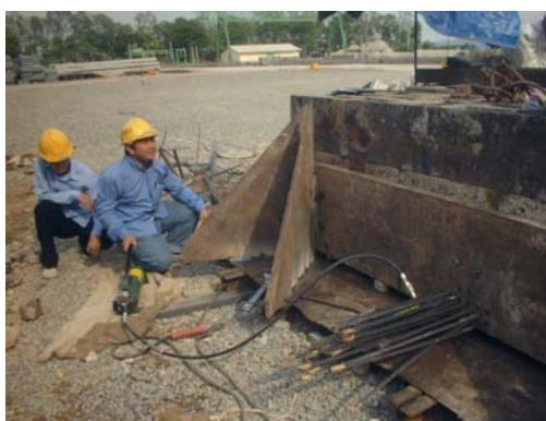
Fig.5.2.4: Tensioning PC strands
