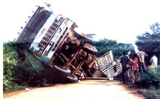
Fig.2.1.3.2 Overloaded truck caused the collapse of a bridge in Mongkul Borei on 07 Sep. 2004
