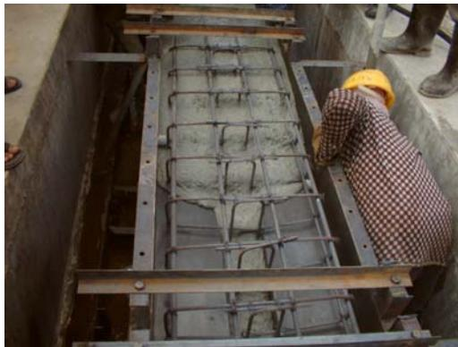
Fig.5.2.6: Casting SCC
