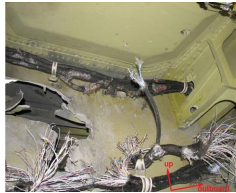
Fig.3 Damage on wiring systems
