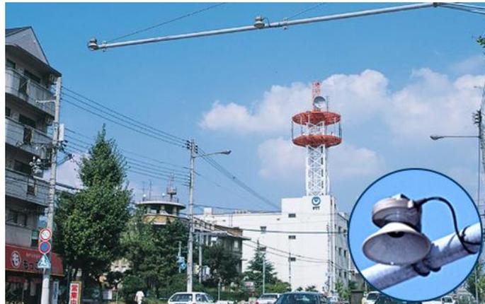
Fig.1-4 Ultrasonic vehicle detector
